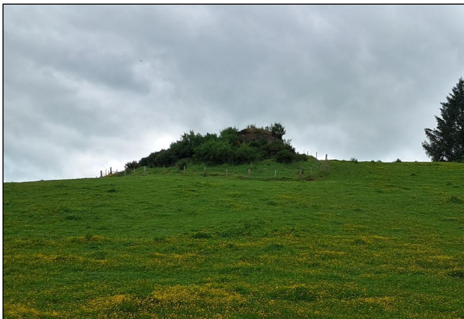
Figure 3.1: View of one of the pillboxes forming part of the Cowie Line, Pillboxes & Anti-tank Blocks NE of Whitehill (Asset 169; a Scheduled Monument), facing south.
