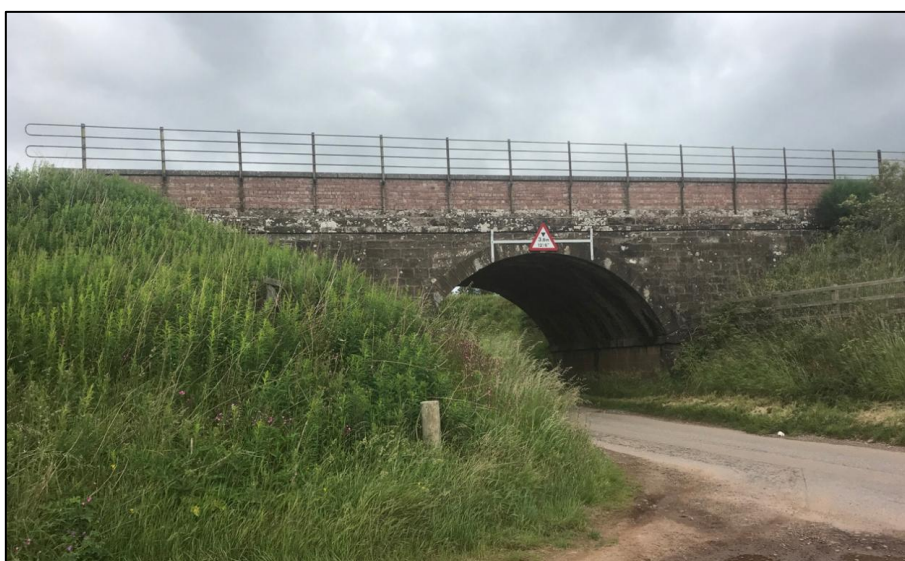
Figure 3.13: View of Mondynes, Railway Bridge (Asset 89), facing north.
